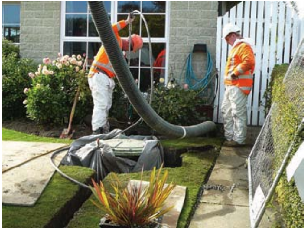
Installation of tank in progress
