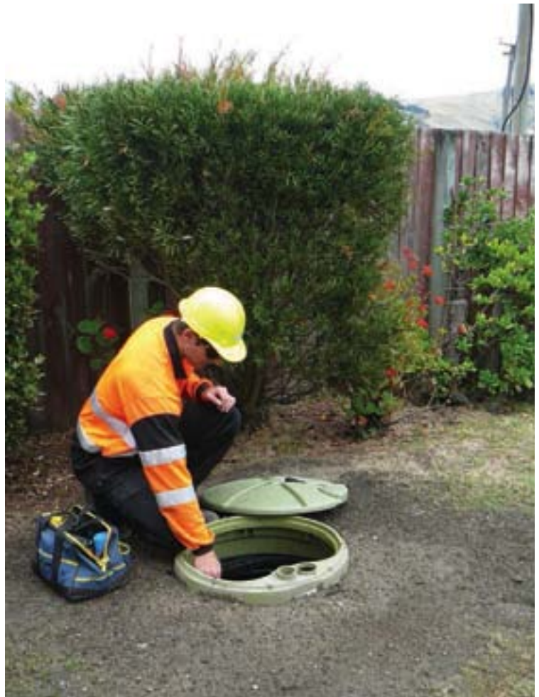
Final inspection of E/One system
